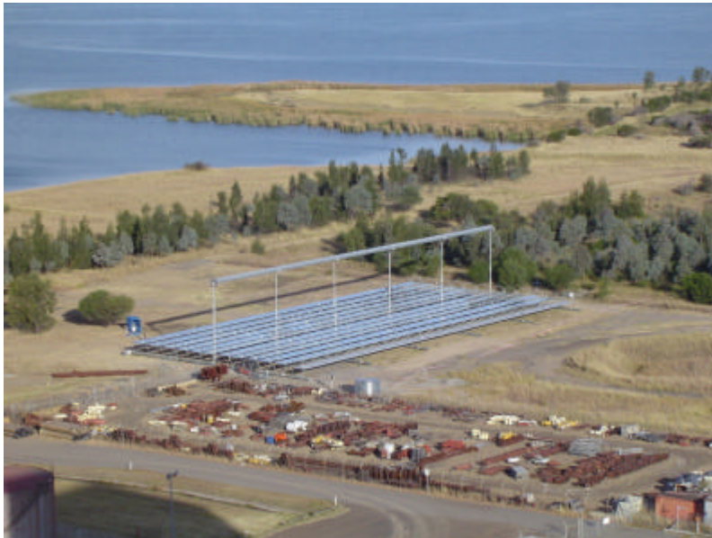
Fig. 1. The 1350 m 2 Stage 1 array and tower line produced by SHP at the Liddell power plant site. This plant will be 100 times larger by stage 3.
